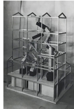
Figure 5 (left): Photograph of draft-tube model. (TVA Structural Model Shop pamphlet 1938)
