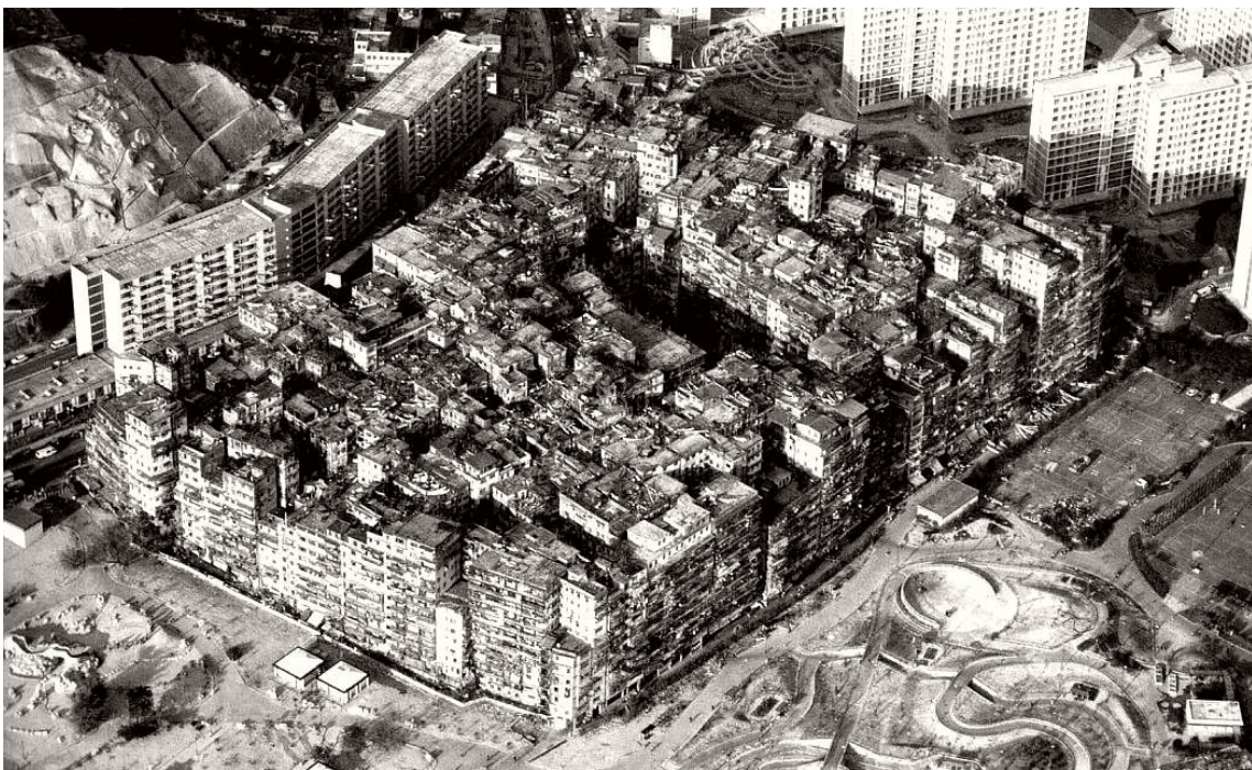
Figure 9: Aerial view of Kowloon highlighting the almost monolithic nature that urban fabric had. (Girard, Lambot, 1993)
