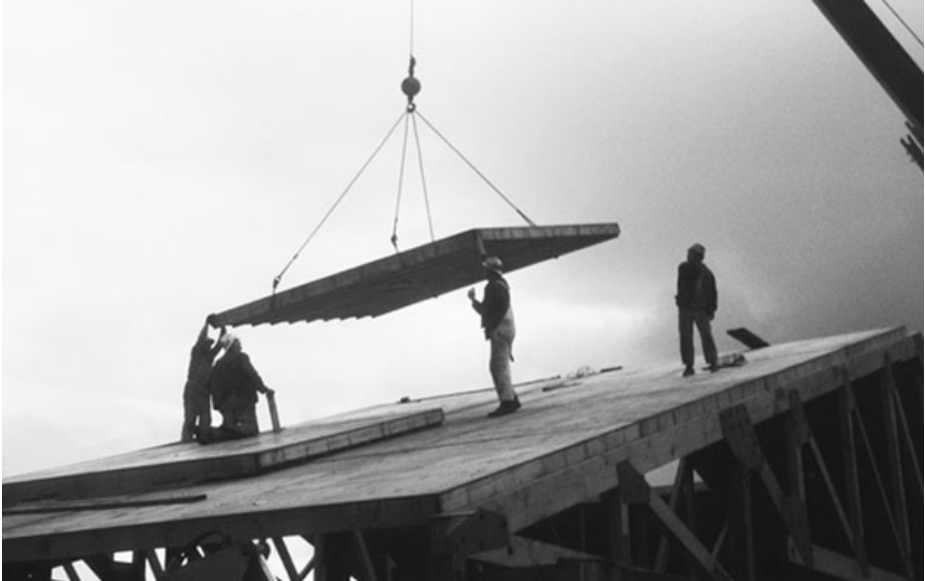
Figure 2: Installing prefabricated SELCO Credit Union building roof panels, 1972. Source: Daniel Herbert
