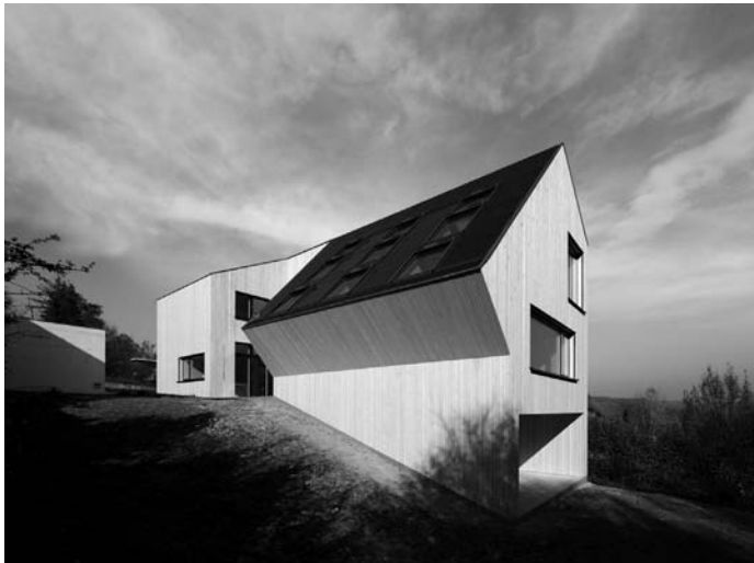
Sunlighthouse, 2010 Pressbaum, Austria New single-family house Picture: Adam Mørk
