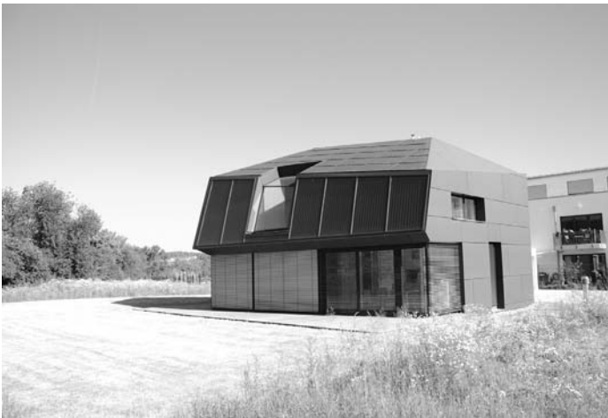
Haus der Zukunft, 2009 Regensburg, Germany New single-family house 175 m 2 Picture: Gitte Gylling
