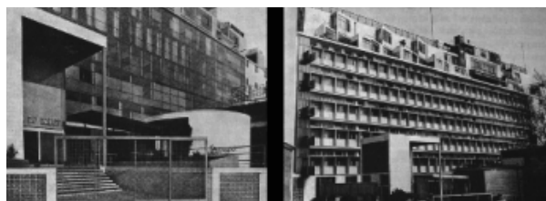
Fig. 2: Le Corbusier's Cite de Refuge: original project (left) and with shades (right), (Banham 1984)
