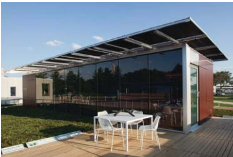
Figure 4 Exterior view of the south Facade of the LivingLight house from the public deck. The glazing appears dark and reflective, contributing to the reading of the glass house as monolithic and private. Cylindrical photovoltaic modules extend over the glazing to provide shade.
